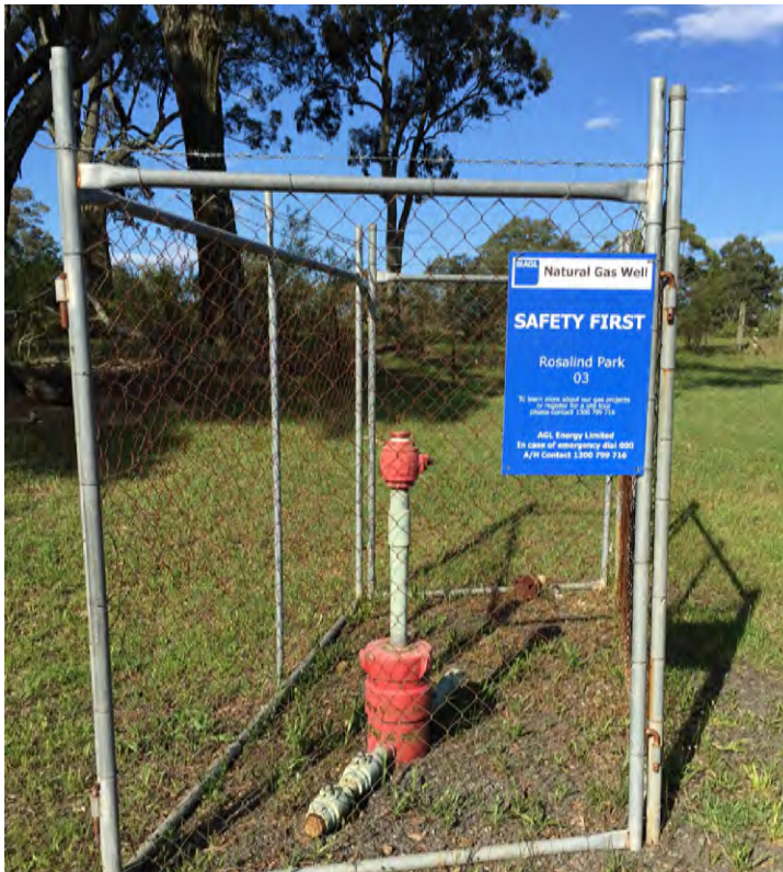
Figure 10 – This photograph of Rosalind Park coal seam gas well No. 3 illustrates the limited extent of infrastructure and local impact associated with a non-operational coal seam gas well
